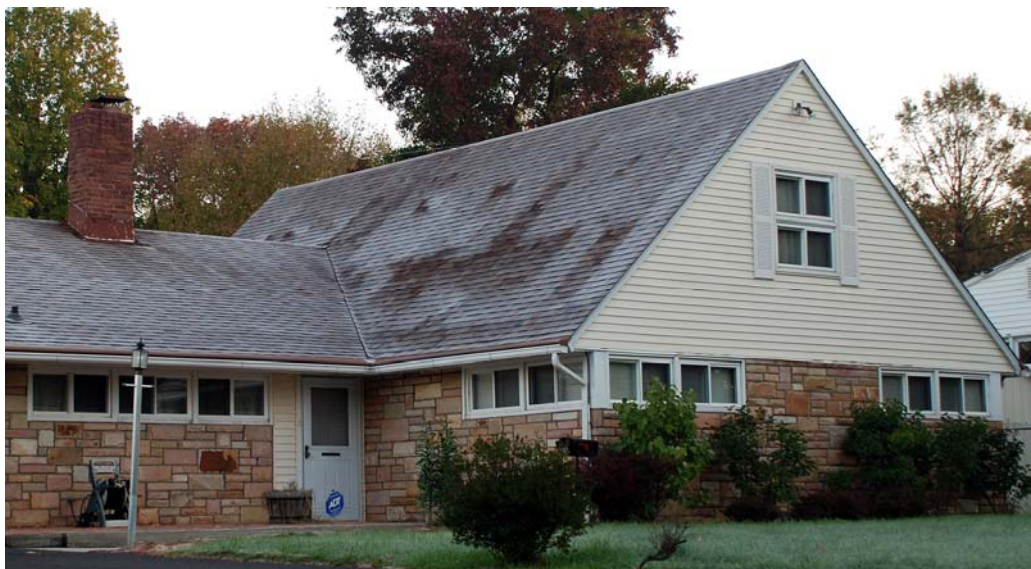
Figure 9: Photo of Levittown roof with heat loss patterns.
