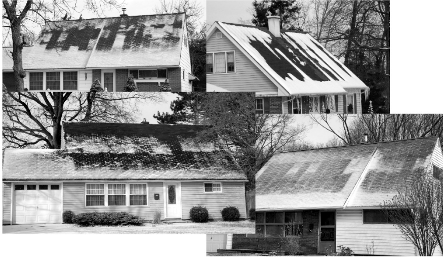
Figure 3: Suspected Insulation Slippage - Levittown PA
